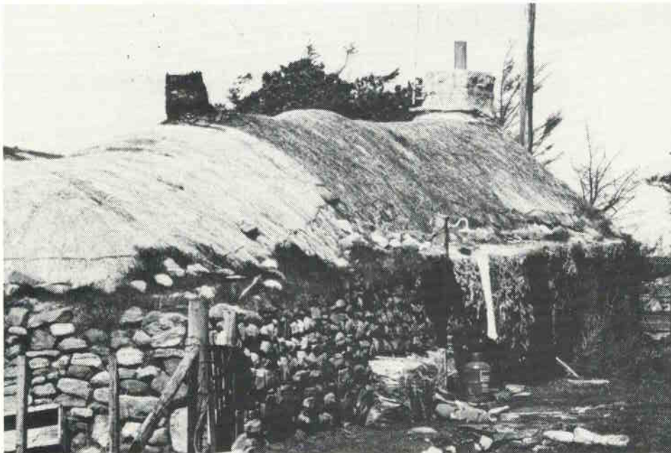
A blackhouse at Callernish, Lewis, with a stone chimney on the right, and a wooden chimney in the middle. The thatch of the byre at the left is lower than the thatch of the house. The wall ledge, tobht , can be clearly
