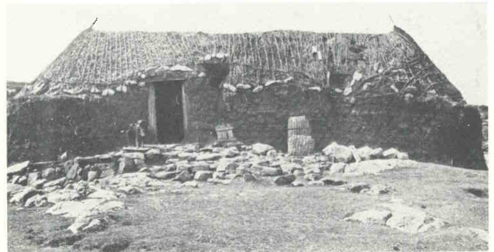
A house built of solid turf at Loch Eynort, South Uist, Inverness-shire.
