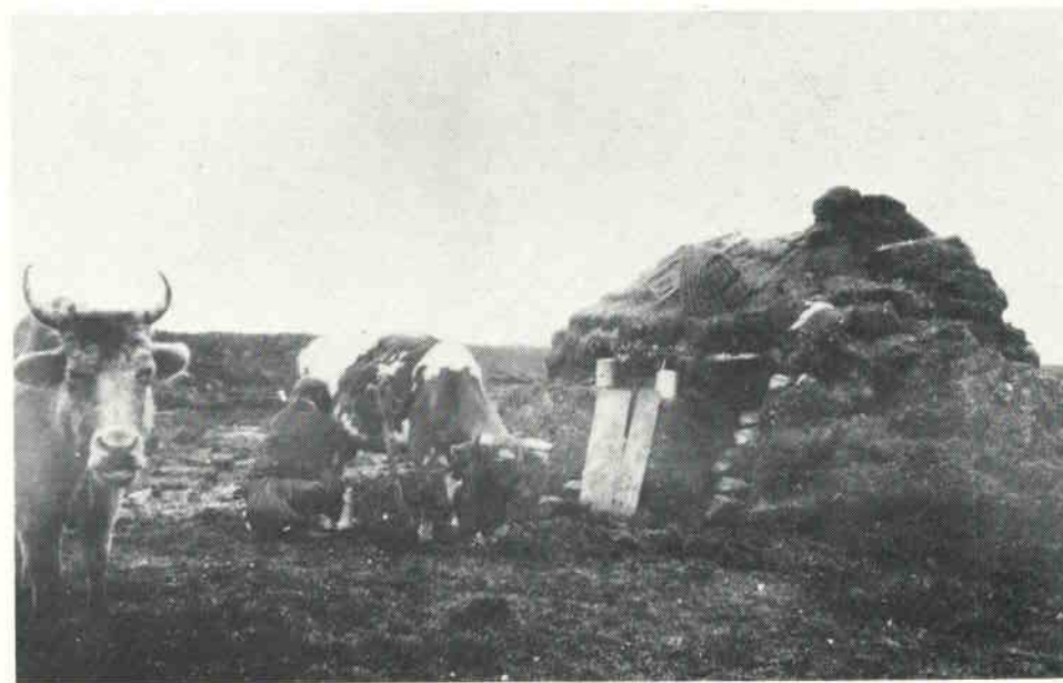
Early morning milking at a Lewis shieling, ante 1928. The stone walls of the hut are covered with turf. C 1228
